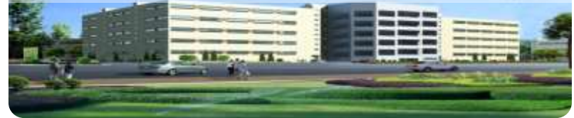
Domestic Logistics Centre (5 floors 83,500 m 2 )
