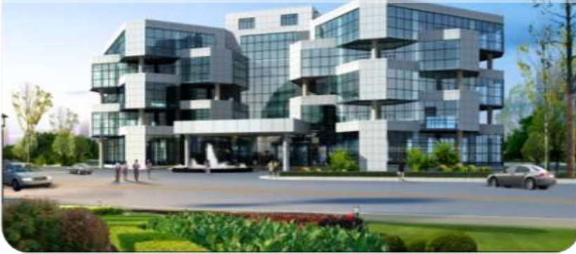
Office. Customs Building (5 floors Twin Tower Total 9,870 m 2 )
