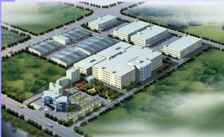
EG Xinsha Port Logistics Centre (500,000 m 2 )
